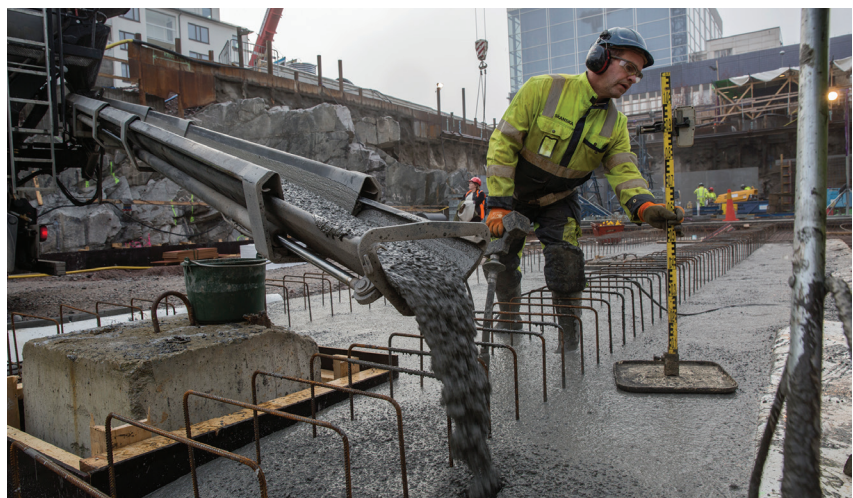
Heavy concrete flows in the same way as standard concrete and can be placed using standard equipment.
