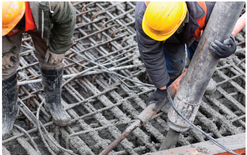
Heavy concrete flows in the same way as standard concrete and can be placed using standard equipment.
