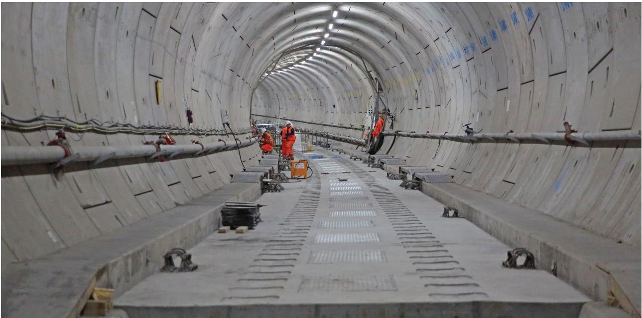
Floating track slab preparation at Tottenham Court Road. Source: ©Crossrail Ltd.
